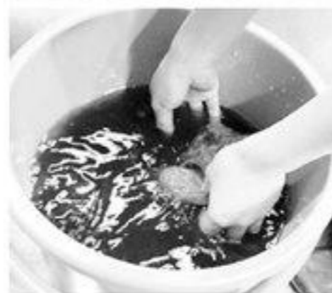
Sludge can be sufficiently removed just by lightly rinsing the filter media in a bucket pre-filled with tank water.
