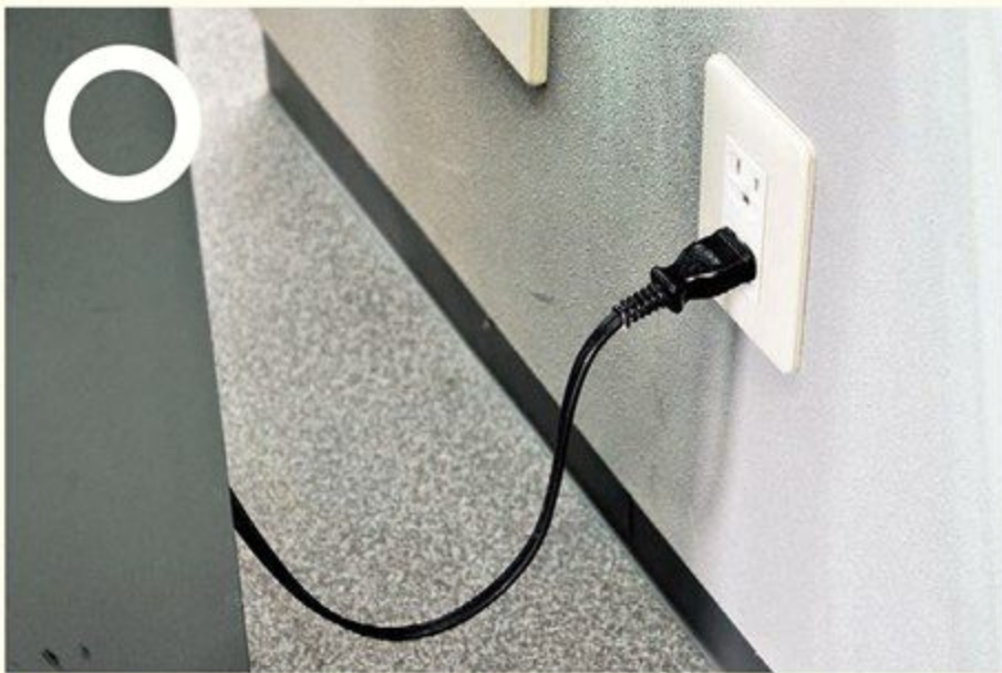
If the cord is sagging, water does not reach the plug even when the water drips along the cord.
