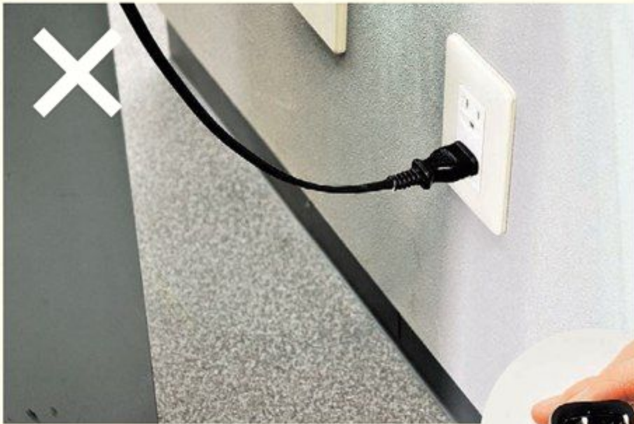
If the cord is tight, dripped water can reach the plug at the receptacle.
