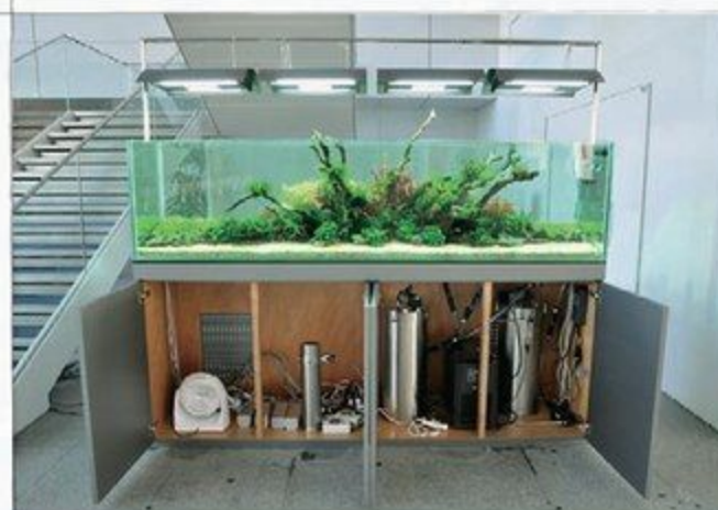
This is how the layout looks after the tank is filled with water and the equipment is all set. Powerful lighting systems and filters are used for this layout. A large chiller and exhaust circulator were also installed to control the rise in water temperature in summer.
